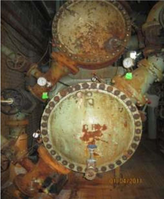
These Heat Exchangers in a power plant are 42" in diameter and have 36 fasteners securing each cover plate. Each metallic cover plate weighs in excess of 1500 lbs.
